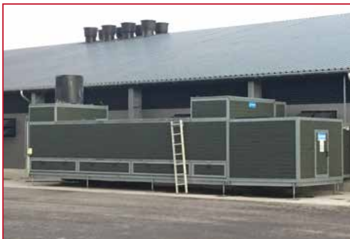
Figure 2.6: Example of a heat exchanger.
