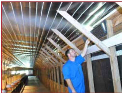
Figure 6.7: Using a smoke test to determine if airflow and operating pressure are correct.
